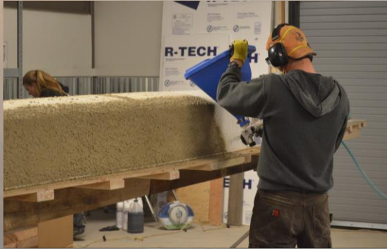
Figure 11: Spraying Concrete Layers
