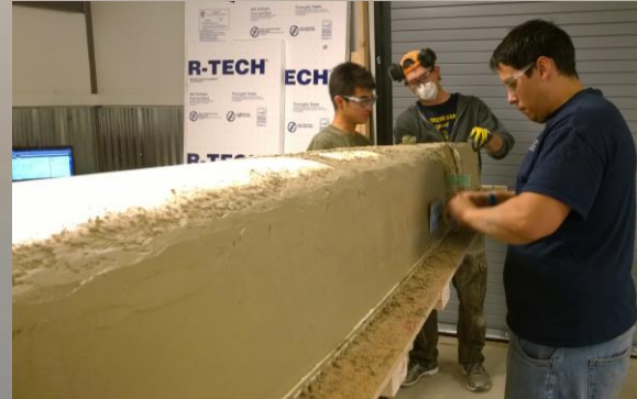
Figure 12: Troweling Concrete Layers
